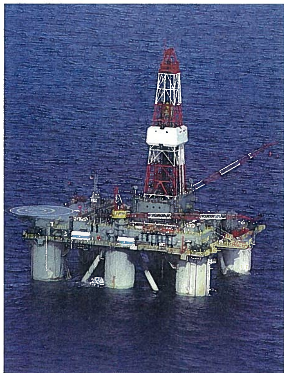
FIGURE 9.13 Offshore Drilling Once the drilling platform is secured to the ocean floor, a number of wells can be sunk to obtain the gas or oil. Source: (line art) American Petroleum Institute.
