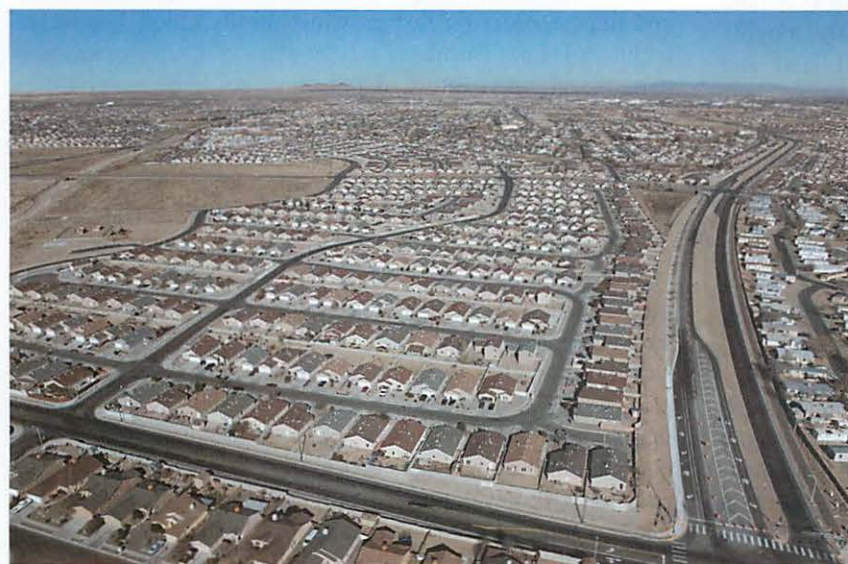
FIGURE 13.5 Sprawl is characterized by the spread of development across large areas of land. This kind of development requires people to drive cars to reach commercial amenities or community centers.
