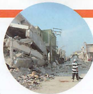
Collapsed buildings in Port-au-Prince, Haiti, following a 7.0 magnitude earthquake in 2010
