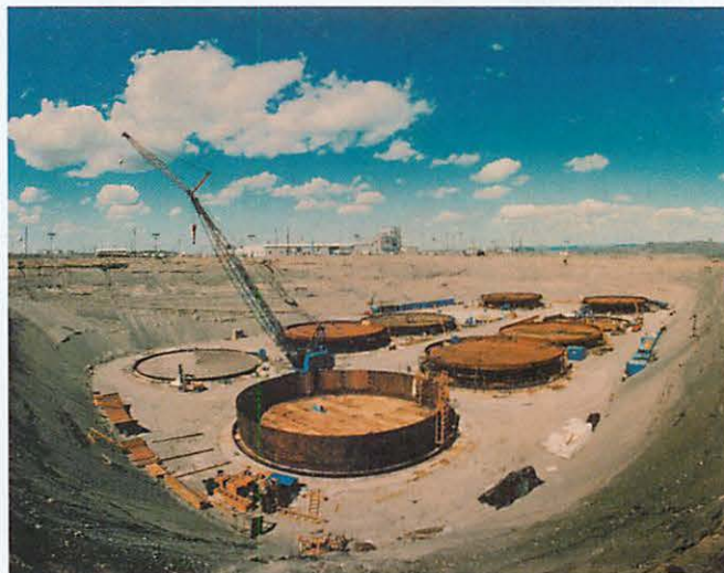
FIGURE 1 Leaks from some of the 177 underground storage tanks at the Hanford Nuclear Reservation in Washington State are threatening to dangerously contaminate the nearby Columbia River.
