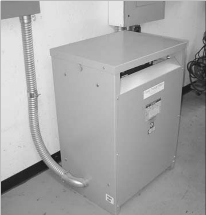
FIGURE 9.16 750 kVA Transformer.
