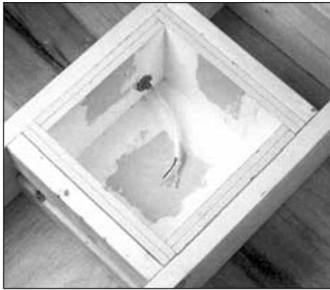
FIGURE 7.36a Recessed lighting enclosure rough-in. (Courtesy Progress Lighting)
