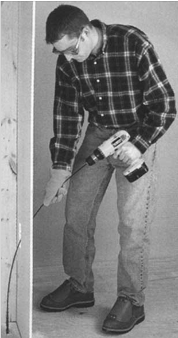
FIGURE 11.2 Flexible drill bits are available in many of styles for a variety of applications, as illustrated in this photo. (Courtesy Ideal Industries )
