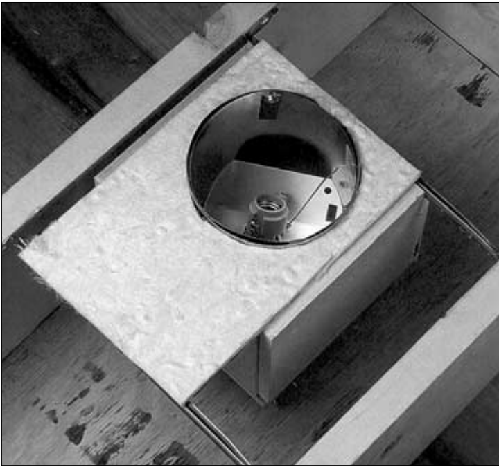
FIGURE 7.37 Self-contained recessed lighting enclosures save labor and extra materials. ( Courtesy Progress Lighting )
