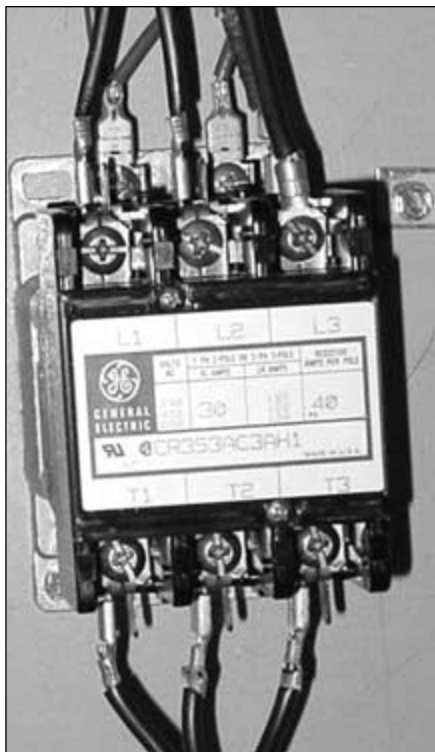
FIGURE 9.21 Three-phase contactor.
