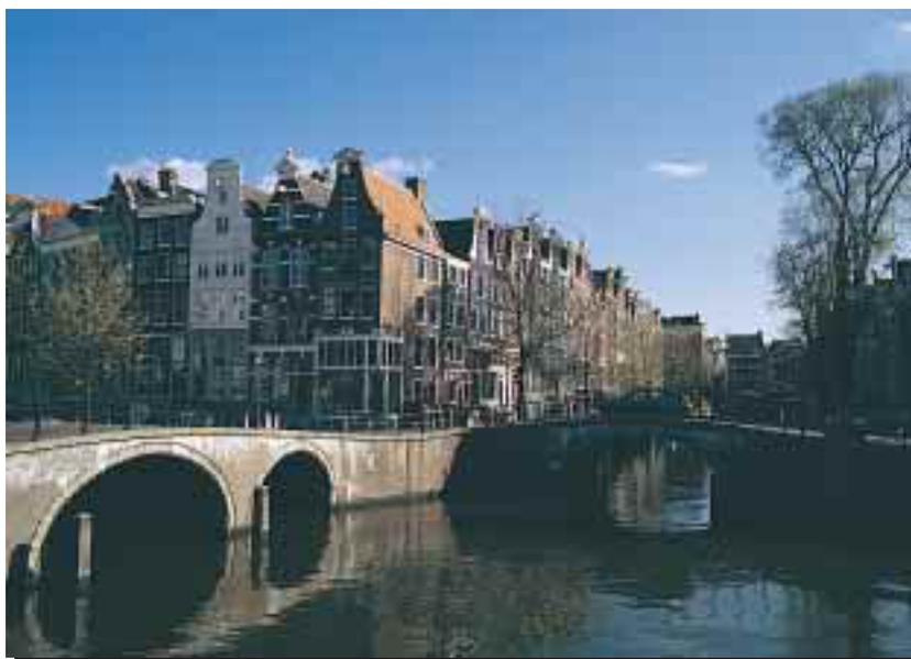
Bridges are often constructed with semi-elliptical arches.
