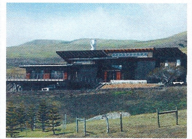
HPA ENERGY LAB
