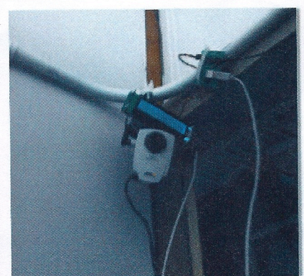
AXIS CAMERA INSTALLATION
